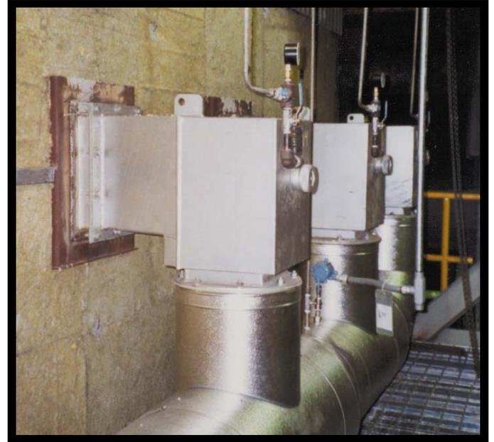
The mill installed a dilute non-condensable gas (DNCG) collection system, also called high volume low concentration (HVLC) NCG, and had identified the No. 3 Power Boiler for disposal of these gases through the boiler's upgraded OFA system. With the OFA system upgrade, the mill had several objectives:
