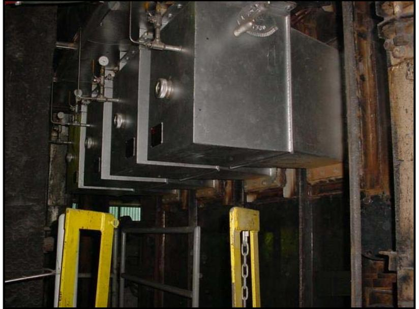
The old overfire air (OFA) system consisted of air ports on the boiler side walls that introduced OFA into the unit in a tangential pattern. A fundamental design limitation that caused insufficient OFA flow capacity and less than optimal mixing of the OFA with the in-flight fuel particles was identified by JANSEN during an in-depth evaluation of the boiler's operation.
