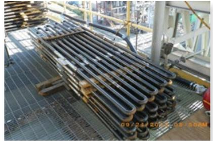
The plant had good experience with Jansen following a successful superheater modification in the CFB Boiler earlier this year. This modification reduced the superheater tube metal temperatures which were limiting the ability of the boiler to operate at higher loads. The photo above shows the superheater tubes ready to be installed in the boiler.
