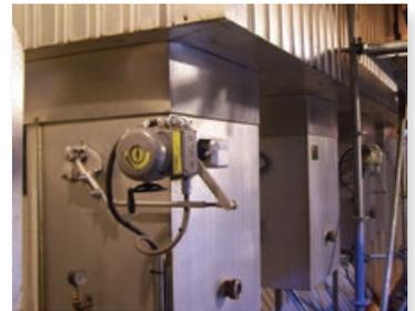
The objective of automatically modulating selected OFA nozzle dampers is to maintain good supply pressure at the OFA nozzles even when flow decreases significantly. The automated dampers adjust to maintain a back pressure in the supply duct so that high jet velocities are maintained through the nozzles with fully open dampers. The result is smooth operation and effective OFA mixing over a wide range of loads.
